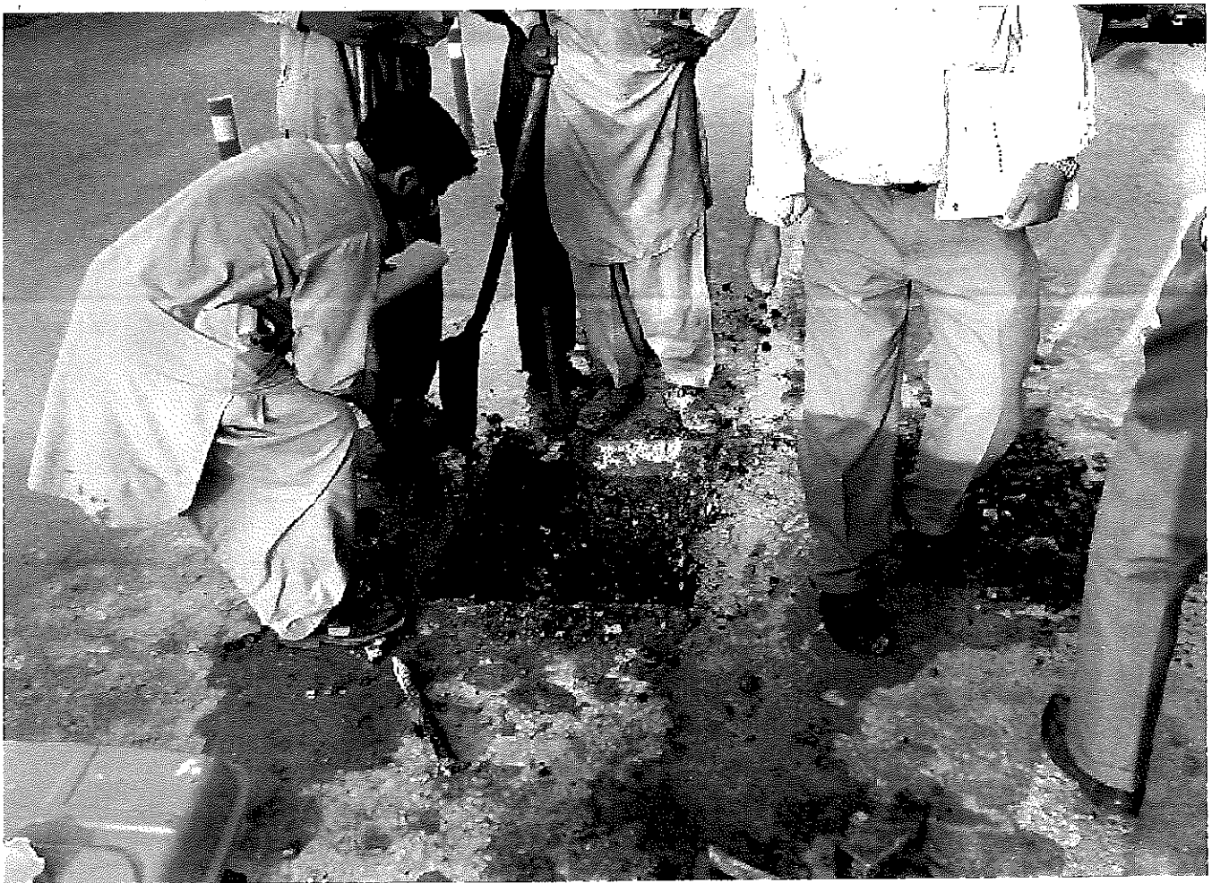
Photo No. 6 DIGGING OF 2' X 2' PIT RD No. 1675+310 Section 7 (N.B)
